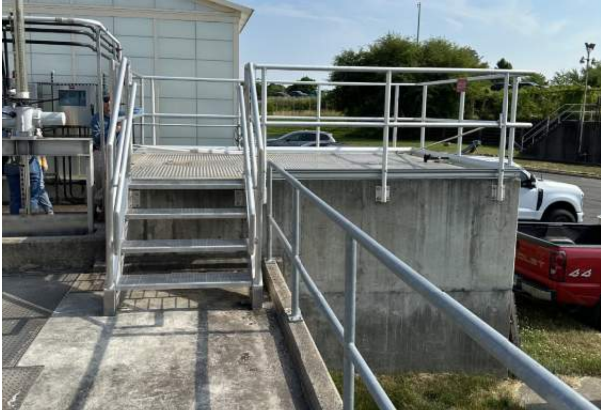
Figure 2.7 Middletown Inlet Box (Southeast corner of the Eastern Detritor)
