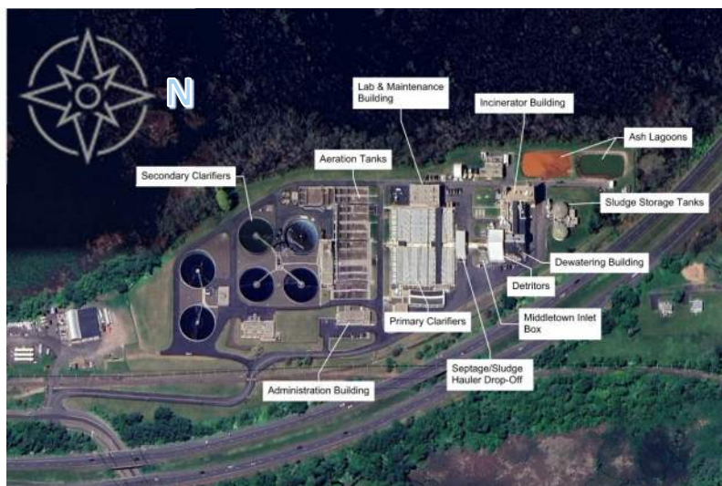
Figure 1.1 Aerial View of the WPCF and Major Buildings/Processes
